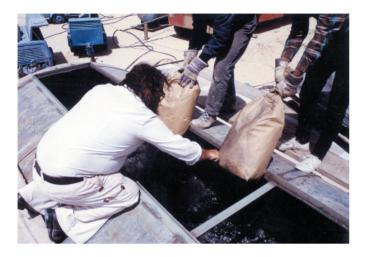
Loresco type SC-2 is a dust-free product and, according to EPA extraction tests, is extremely pure and complies with regulations governing buried products. SC-2 mixes easily with water and may be pumped into deep anode systems. Loresco SC-2 is designed to promote electronic flow between the anode surface and itself.
