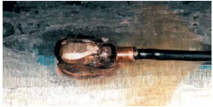
Equipment for copper conductors to steel pipe connections
